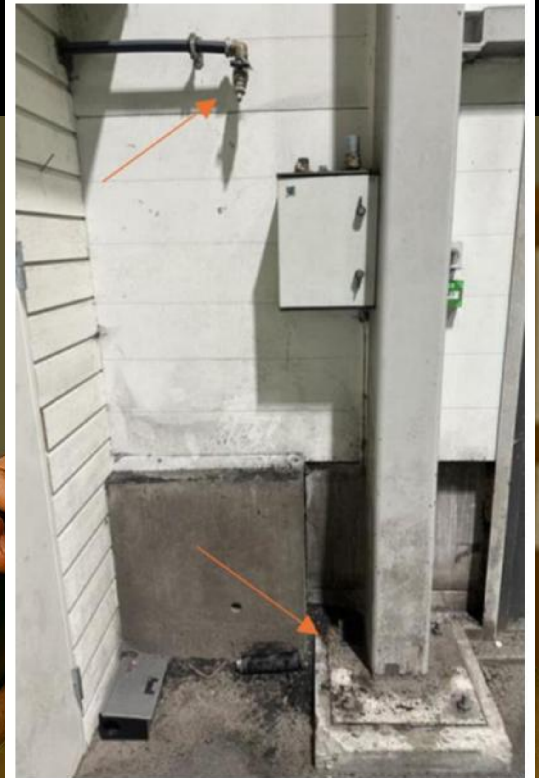
FIGURE 2 | The water faucet used to fill up the truck used to sprinkle the pitch with water before matches, and the crumbed rubber on the floor underneath.
